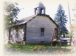
Replica log church, one of the 14 Historical Village buildings.
